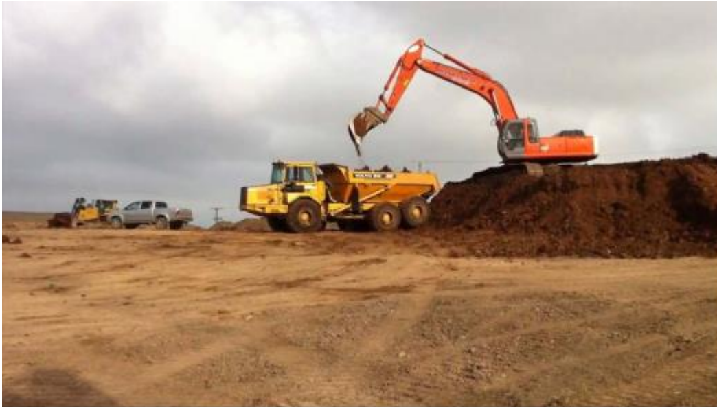
Excavation progress monitoring
